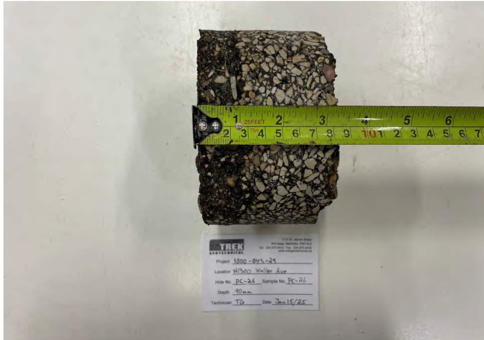
Photo 1: Pavement Core Sample at PC25-26
