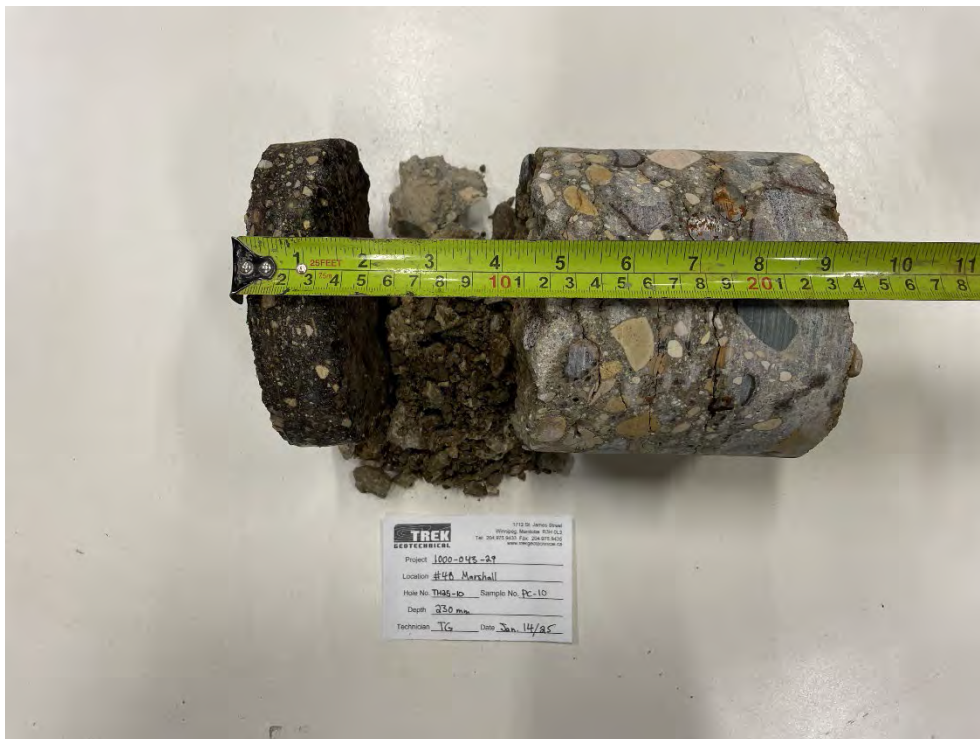
Photo 4: Pavement Core Sample at TH25-10
