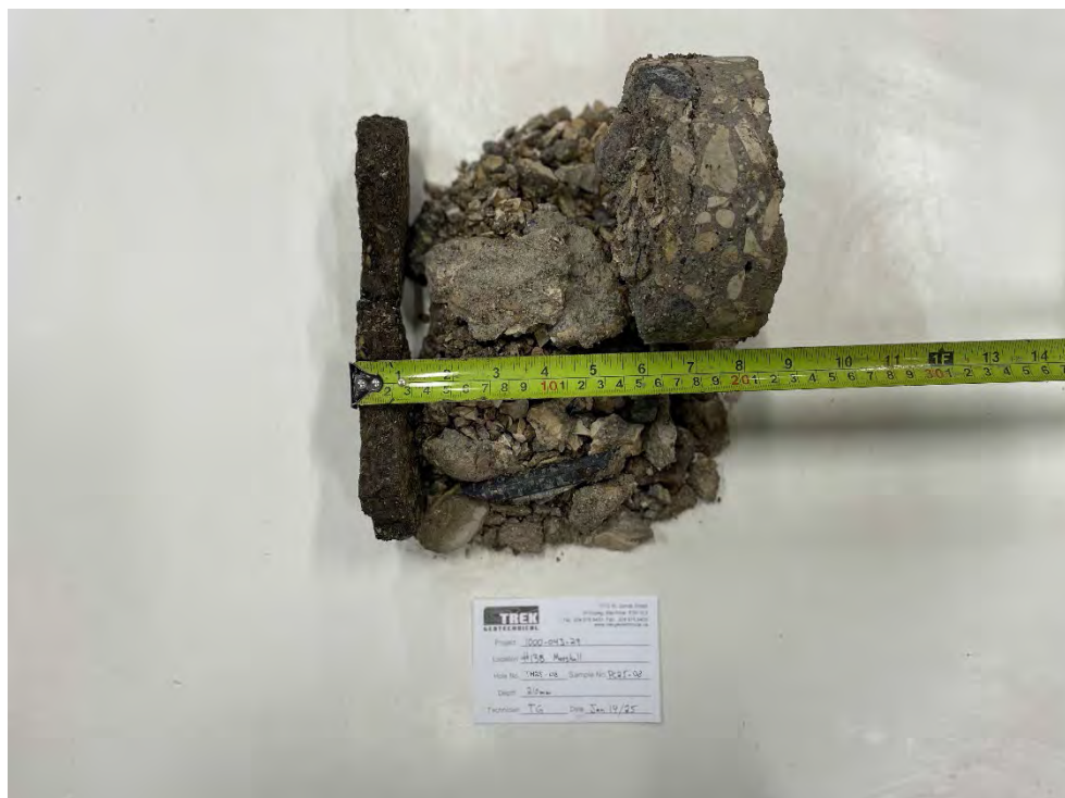
Photo 2: Pavement Core Sample at TH25-08
