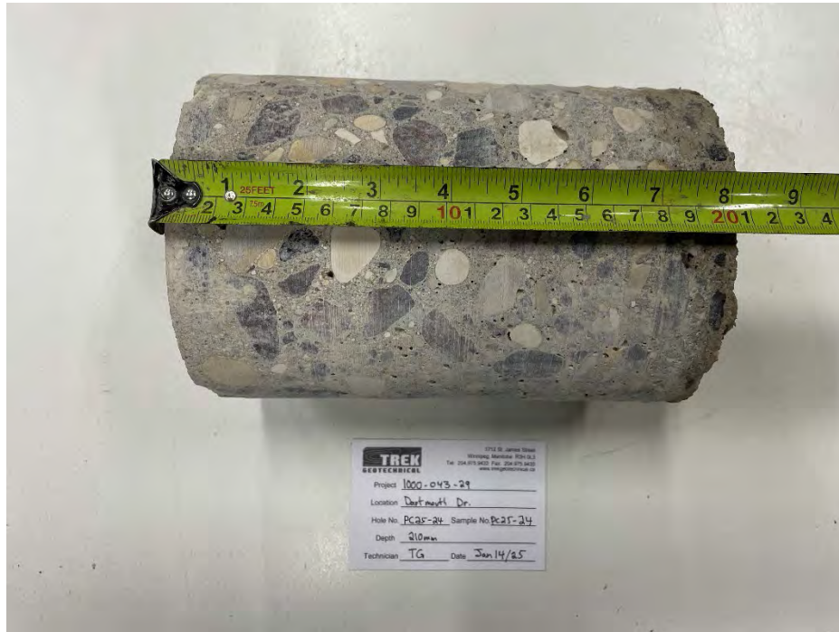
Photo 1: Pavement Core Sample at TH25-24
